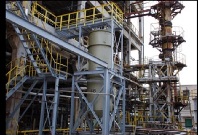
(Top) Steel equipments framework.
